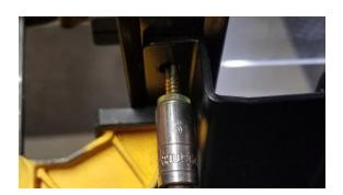
**Step 3**: Using a 8mm socket & drill, install the remaining self-tapping screws.
